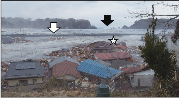
Fig. 1. Tsunami in Taro district on March 11, 2011. Huge tsunami overcame the 10 m height embankment (white arrow) and destroyed the center of the district repeatedly. Next tsunami followed (black arrow). Ms. X was found under the rubble at the white star area. This image reproduced with permissions from Mr. T. Torii.
